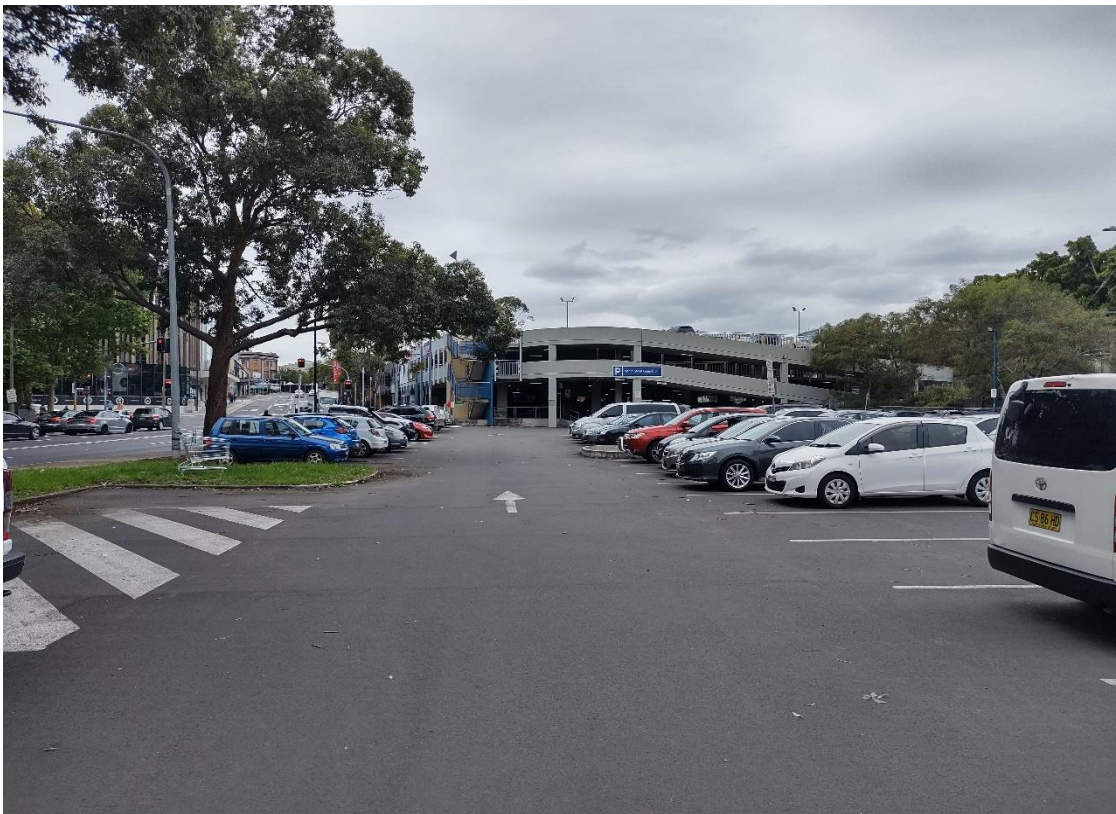
Photo 2: Road level portion of carpark with entrance to multi-storey carpark, facing east
