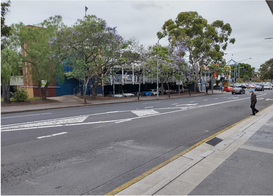
Photo 1: Multi-storey carpark from Marion Street, facing south-west
